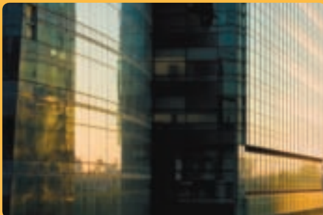
Black Fan Research Center, Boston: Meticulous planning and extensive experience with high-performance built environments enabled EMCOR to construct, within a congested urban area and on a very tight time schedule, 6,600 tons of chillers, 8.5 miles of piping, and 12 custom air-handling units for this state-of-the-art research facility.
